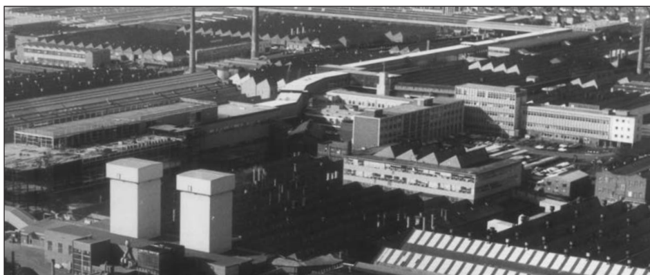
Fig 18 The Cowley Works in 1974 showing the conveyor across the bypass linking the former Pressed Steel and Morris factories
